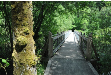
Pedestrian bridge through the Tacoma Nature Center
