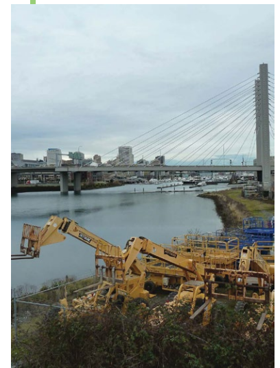
Remediation of heavy metals on the future Waterway Park site
