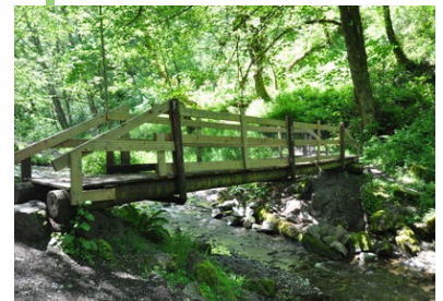
Canopy (top) and pedestrian bridge (bottom) at Swan Creek Park
